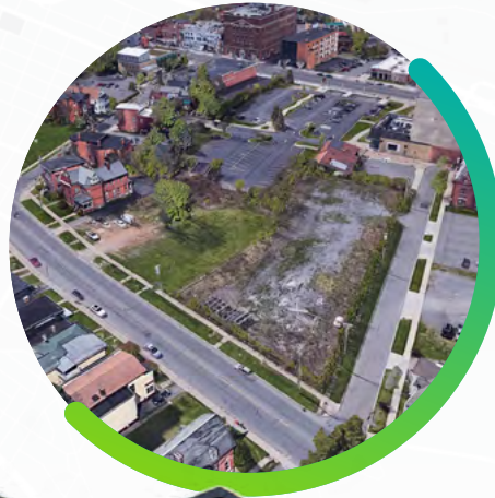
Aerial view of Artspace Utica site
