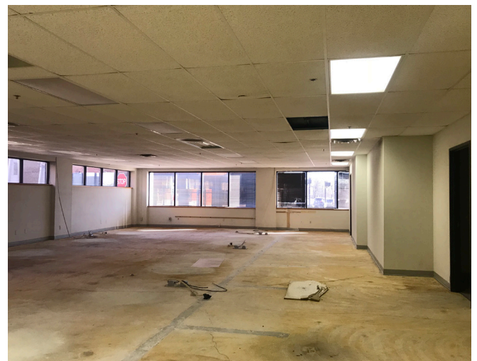
Office Building at 85 North Main Street
