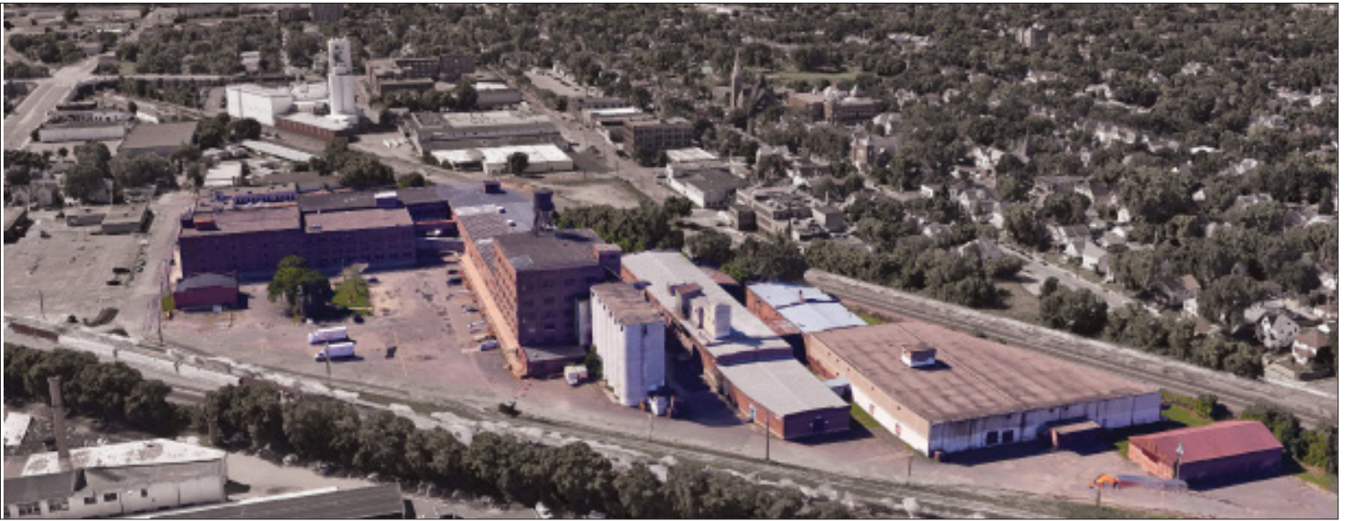
Above: The Northrup King complex, courtesy of the Cunningham Group. The campus is comprised of 13 buildings, with six occupied and seven vacant.
