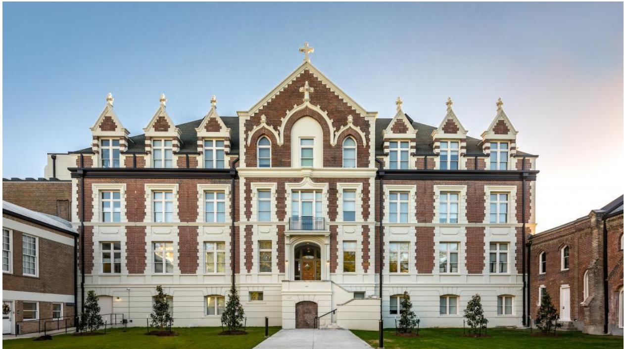
Bell Artspace Campus, New Orleans, Louisiana. This campus had anchored the Tremé neighborhood for over 100 years but sat abandoned after Hurricane Katrina. The Bell Artspace Campus transformed the three largest buildings into 79 units of affordable live/work housing for low- to moderate-income artists, cultural workers, and families. The project also reestablished common spaces for creative use by the residents and commercial tenants. It received the 2019 Advisory Council on Historic Preservation (ACHP)/ U.S. Department of Housing and Urban Development (HUD) Secretary's Award for Excellence in Historic Preservation
