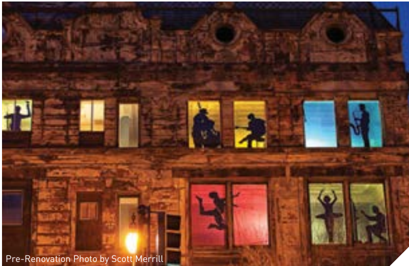
Pre-Renovation Photo by Scott Merrill
